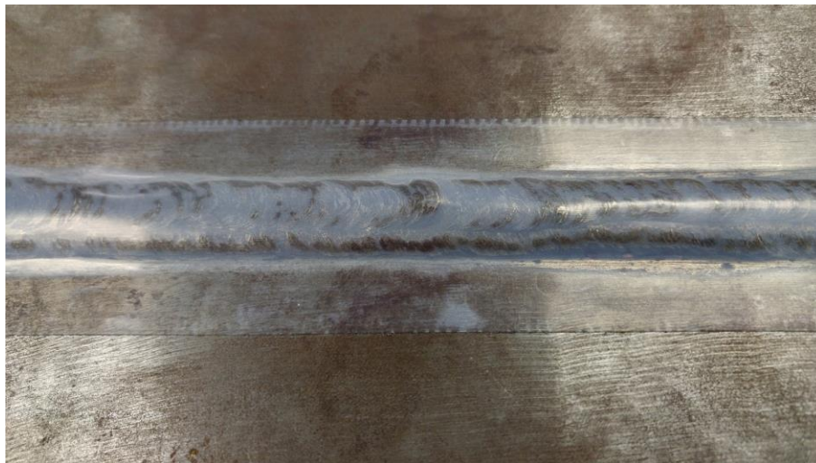
Figure 27. Protective tape applied directly on weld
