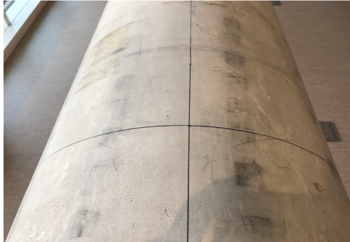
Figure 40: The X and Y datum lines should be defined prior to beginning an inspection
