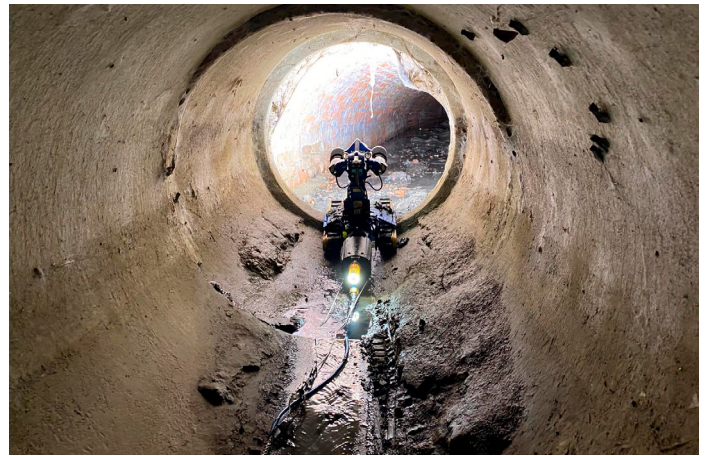
Figure 2: Remote internal pipeline inspection
