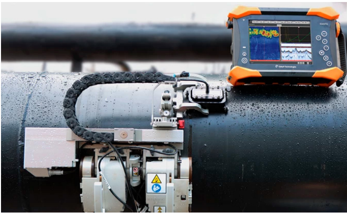
Figure 7: PAUT corrosion mapping with Nav2 and Mantis.
