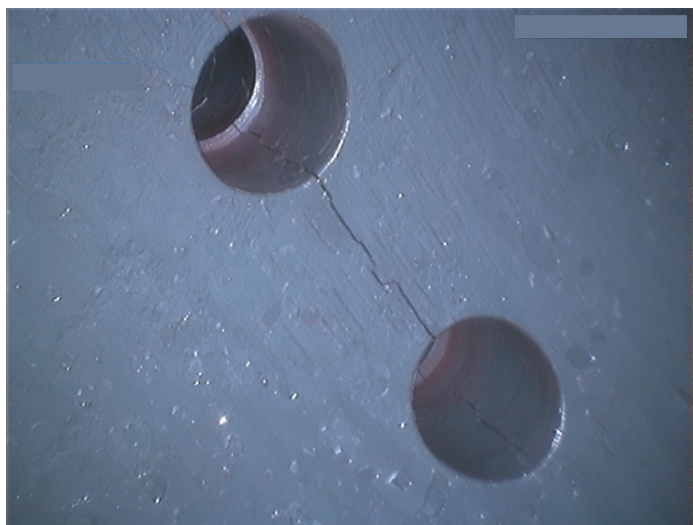
Figure 8: Ligament cracks observed using the Hi-Def PTZx camera.
