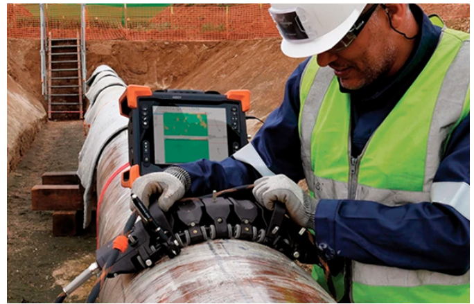
Figure 4: Ditch pipeline inspection using Sypne™ paired with Reddy.
