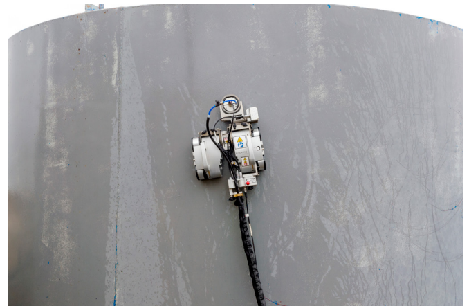
Figure 3: One-axis corrosion scanning.
