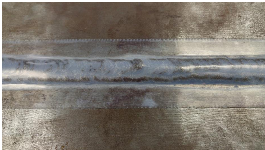
Figure 28. Protective tape applied directly on weld
