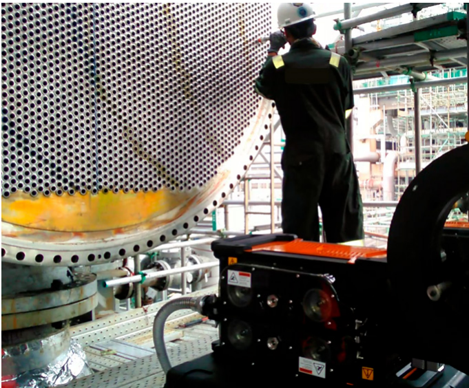
Figure 3: Heat exchanger inspection using the Probot.
