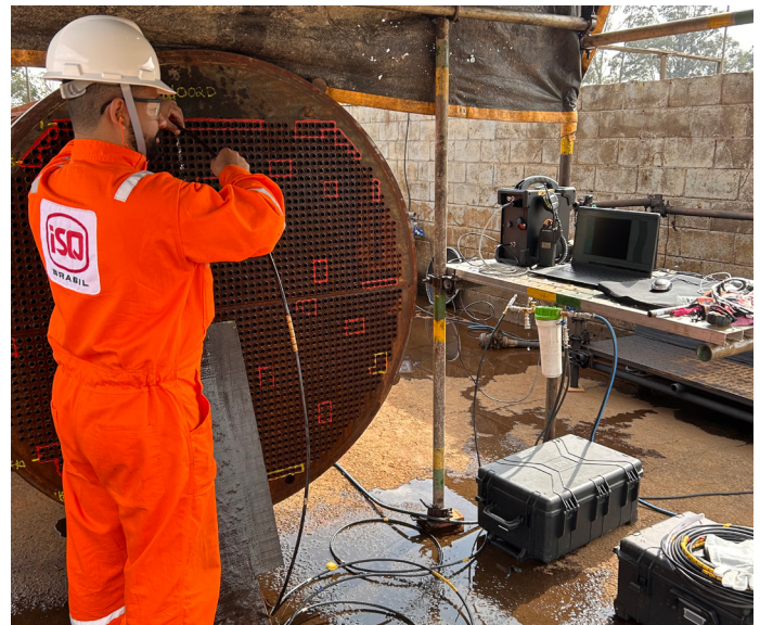
Figure 4: Heat exchanger inspection using the internal rotary inspection system (IRIS) with Ectane 3.
