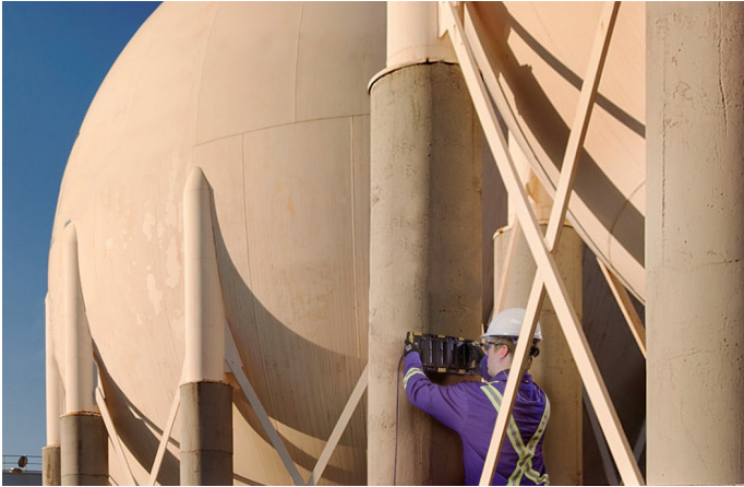
Figure 1: Sphere legs inspection with PECA.
